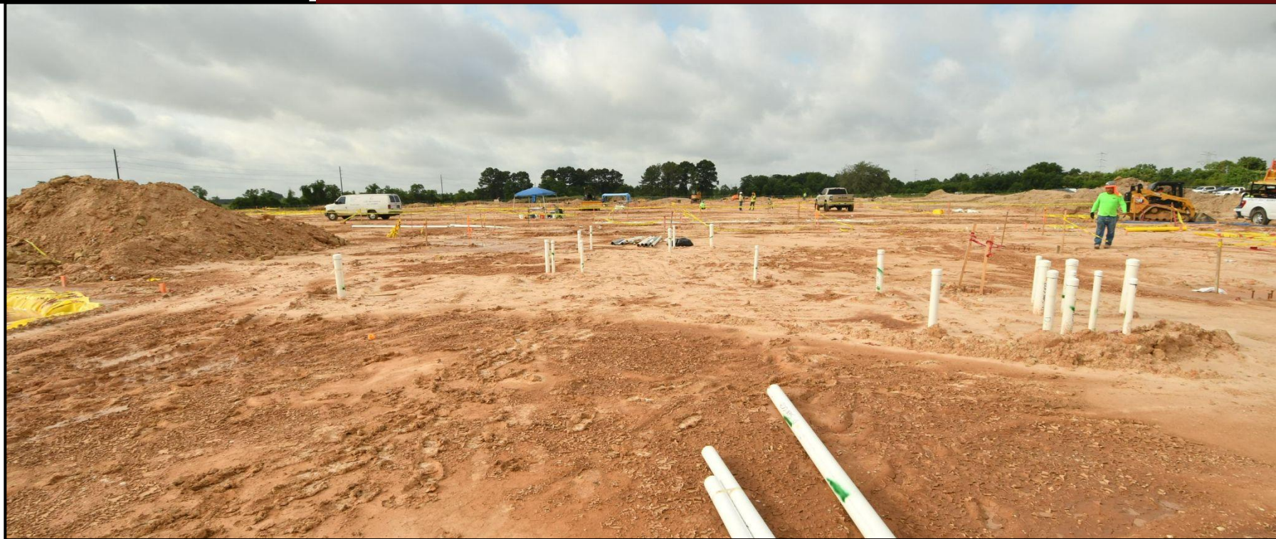
Subfloor Plumbing in Progress
