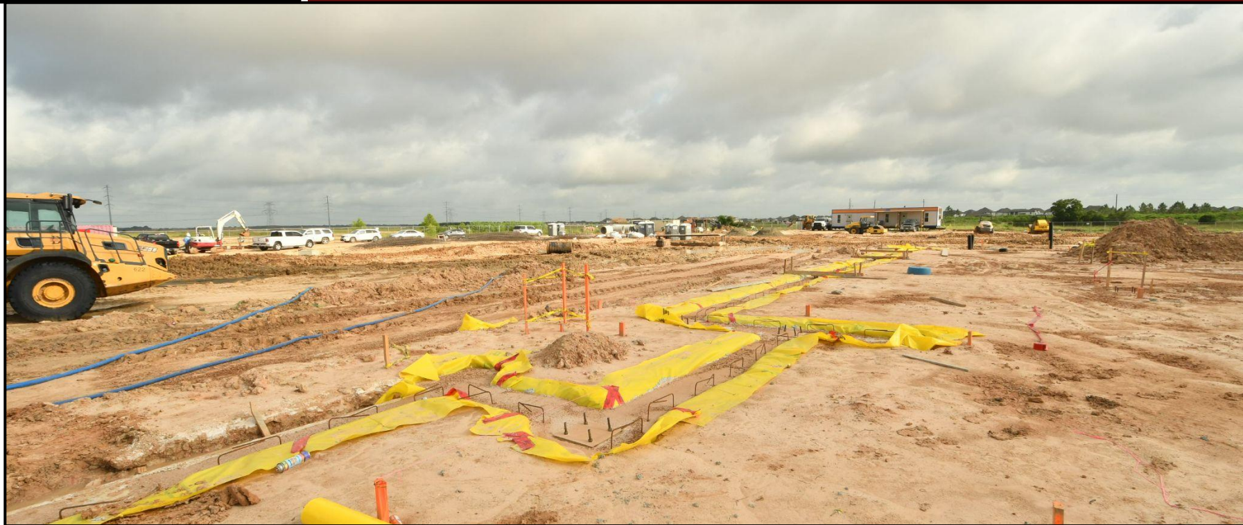
Grade Beam Foundations in progress
